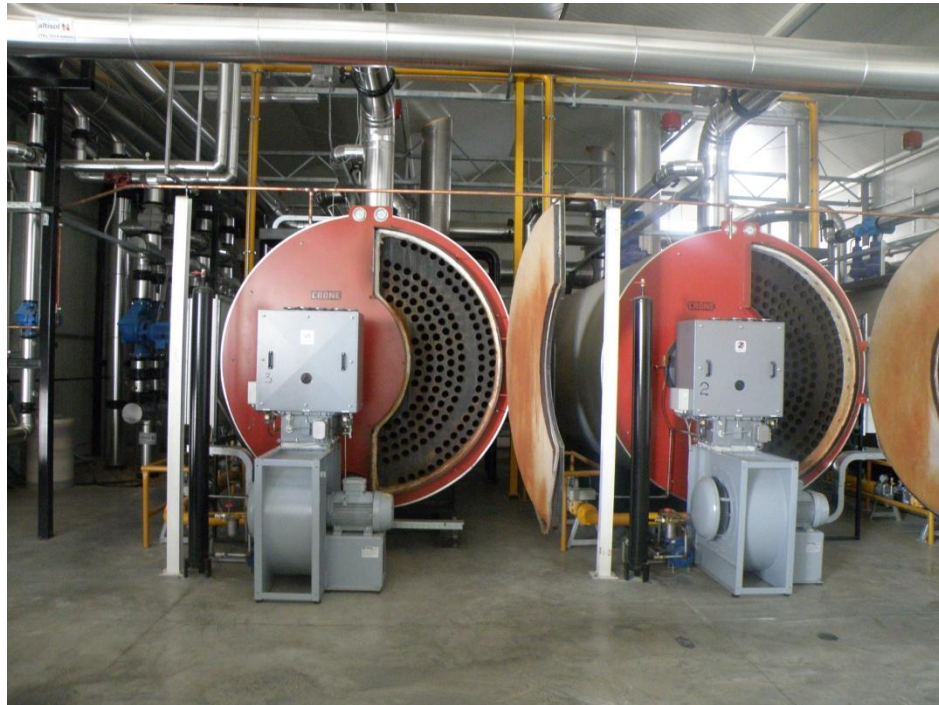
Central warm water boiler
