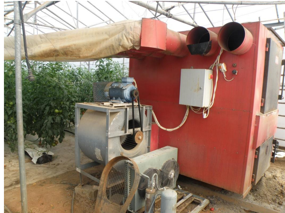
Directly fired air heater
