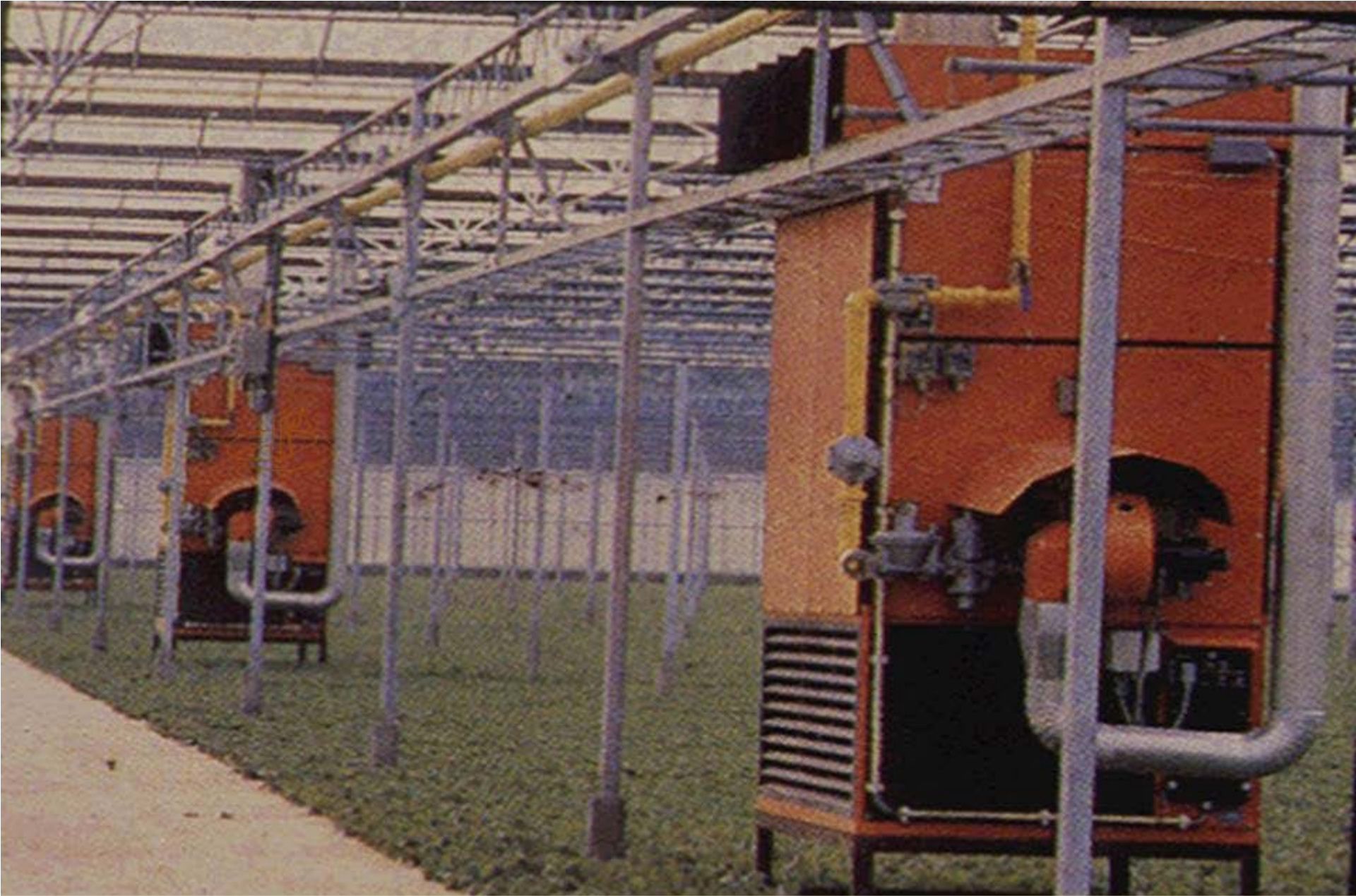
Air heaters suitable greenhouse heating
