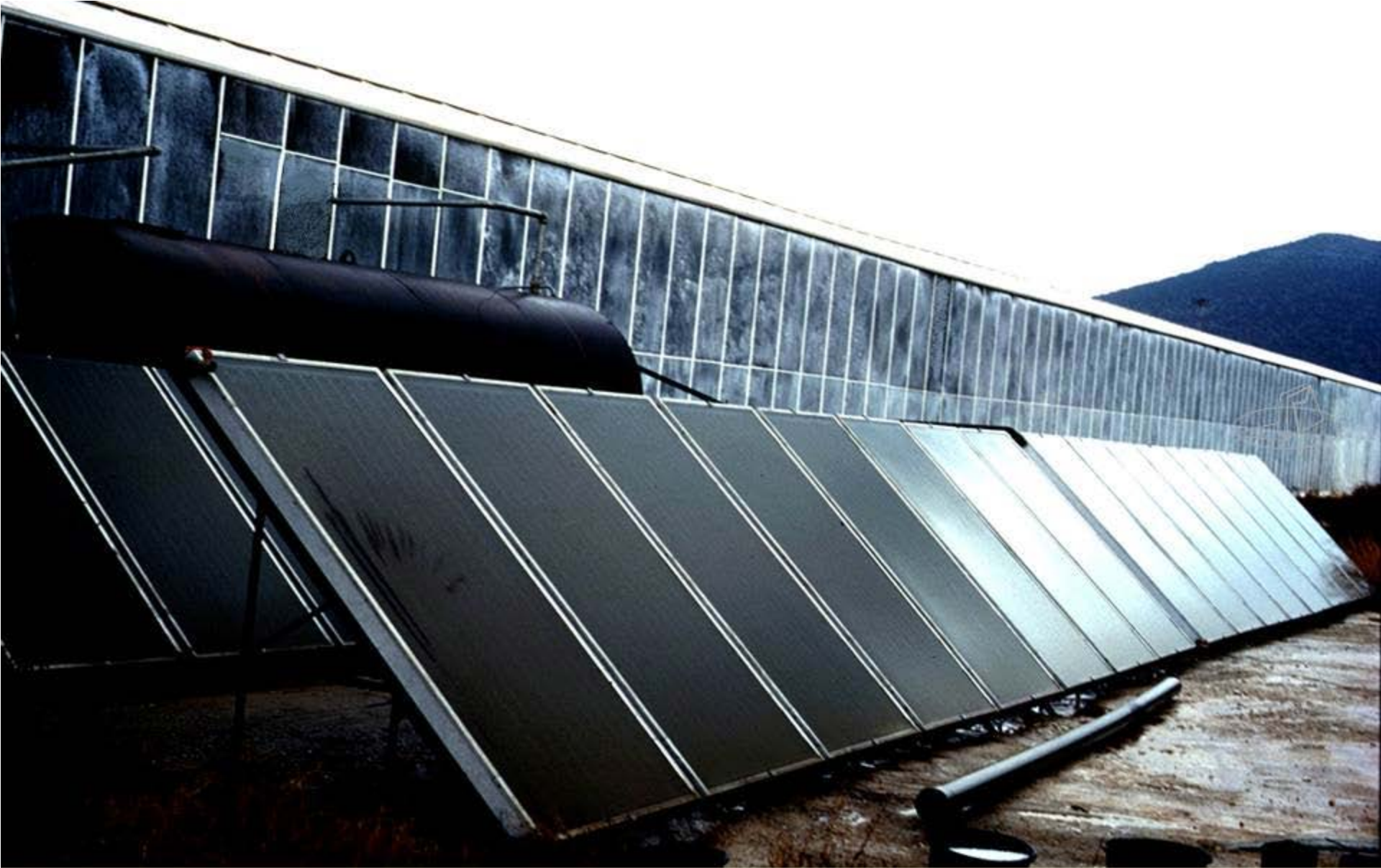
Solar collector, hot water industrial type, for greenhouse heating
